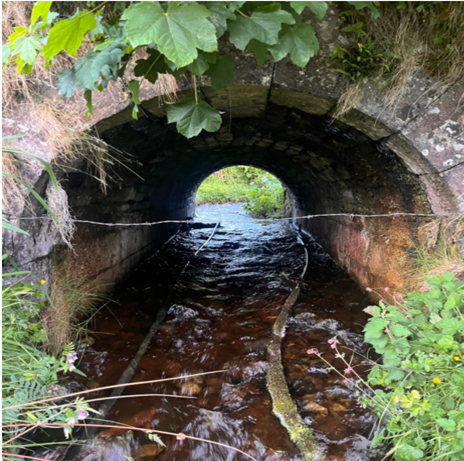
Figure 2.4 Bridge R282-4 under R282 with omitted watercourse.
